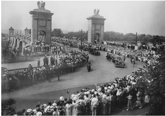
FDR crosses the Market St. Bridge 21
